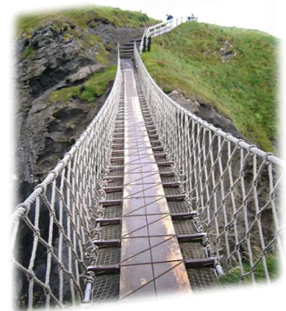
Carrick-a-Rede Rope Bridge - most na linach.Str. 6
